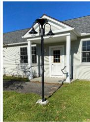
approximately 2,190 Kilowatt hours per year at an approximate cost of \$438.25. It is our expectation is that the new lamps will have a lifespan of 10 years at a total cost savings of \$4,380. The solar lamp structure was chosen to be consistent with the Town Plan to provide aesthetically pleasing lamps that are consistent with the Town's historical school street and train depot building.
